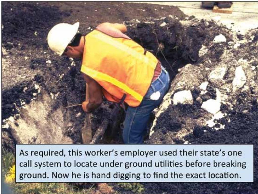
As required, this worker's employer used their state's one call system to locate underground utilities before breaking ground. Now he is hand digging to find the exact location.
