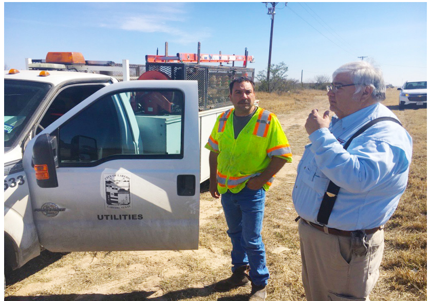
Juan Vasquez (right), TEEX WWW Instructor II, provides operational assistance to City of Laredo utilities professionals during water main repairs. (Photo by Steve Ash)
